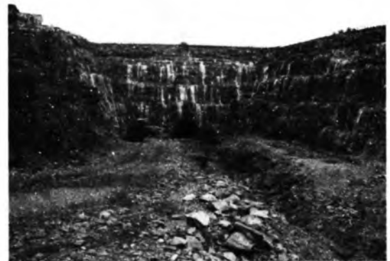
Photo 3: Outlet Portal of the Bansagar Feeder Tunnel.
