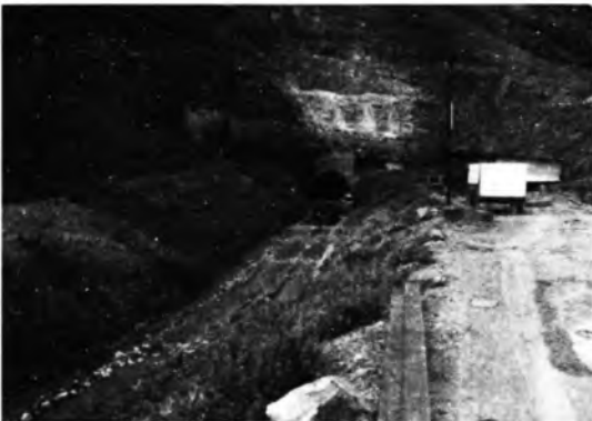
Photo 2: Inlet Portal of the Bansagar Feeder Tunnel.
